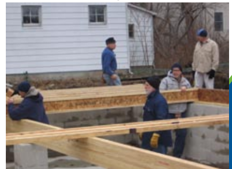
Volunteers lay beams on the foundation of the new house.
